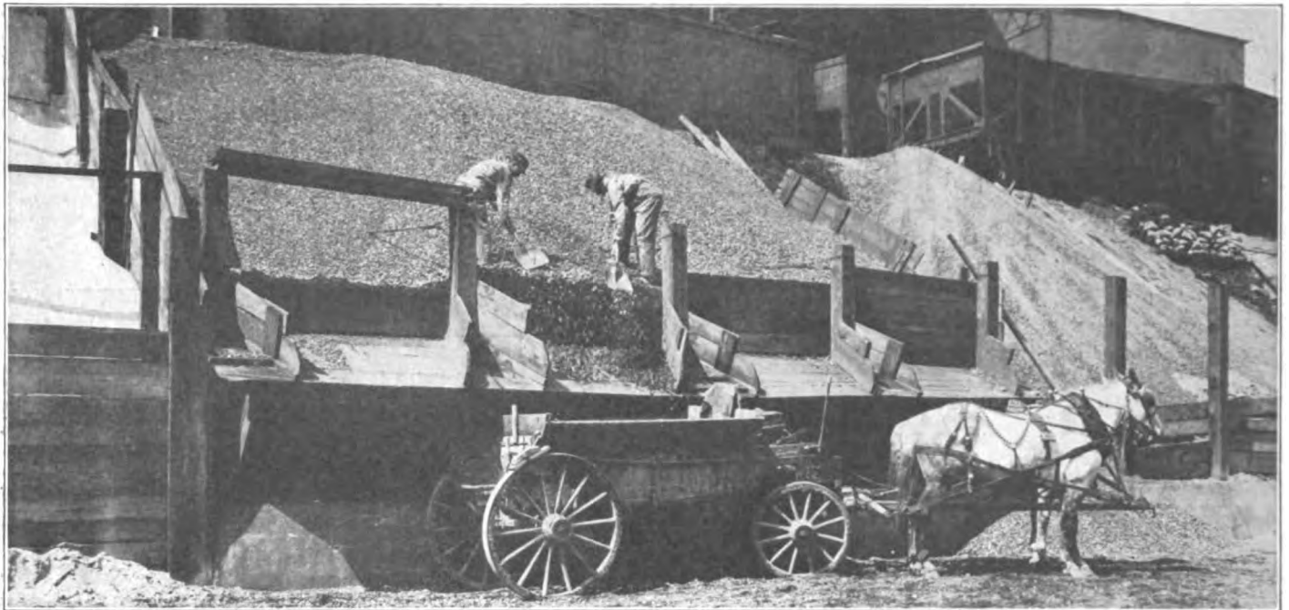
With only a slight amount of shoveling, bulk materials are loaded from stock piles to wagons.
