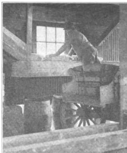
Cement and lime are stored on the second floor and chuted through any one of four trap doors to a loading platform on the ground floor. Materials are also chuted from cars to warehouse, as shown in the diagram above, thus using gravity to reduce the cost of handling materials
