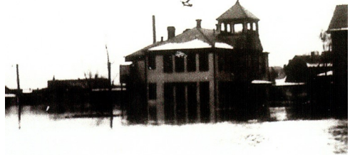
A rare photo of the Loveland School taken during the 1936 flood.
