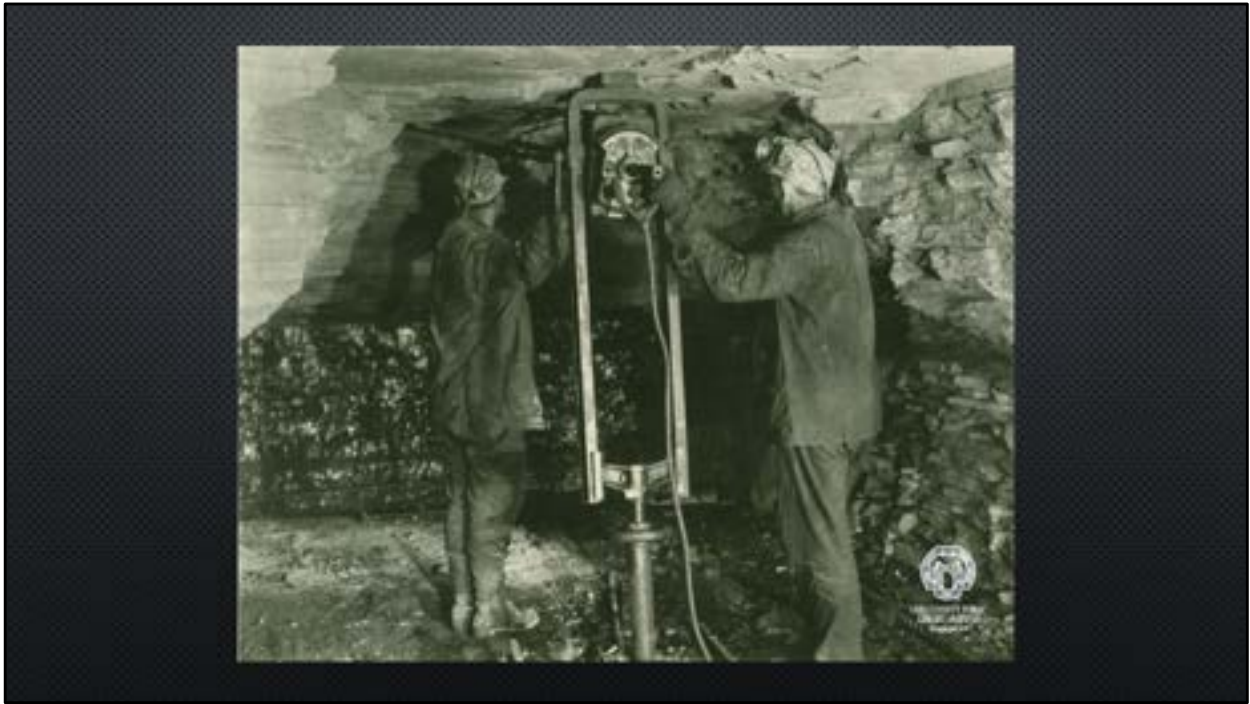
Here are 2 miners drilling the wall for blasting in Steubenville.
