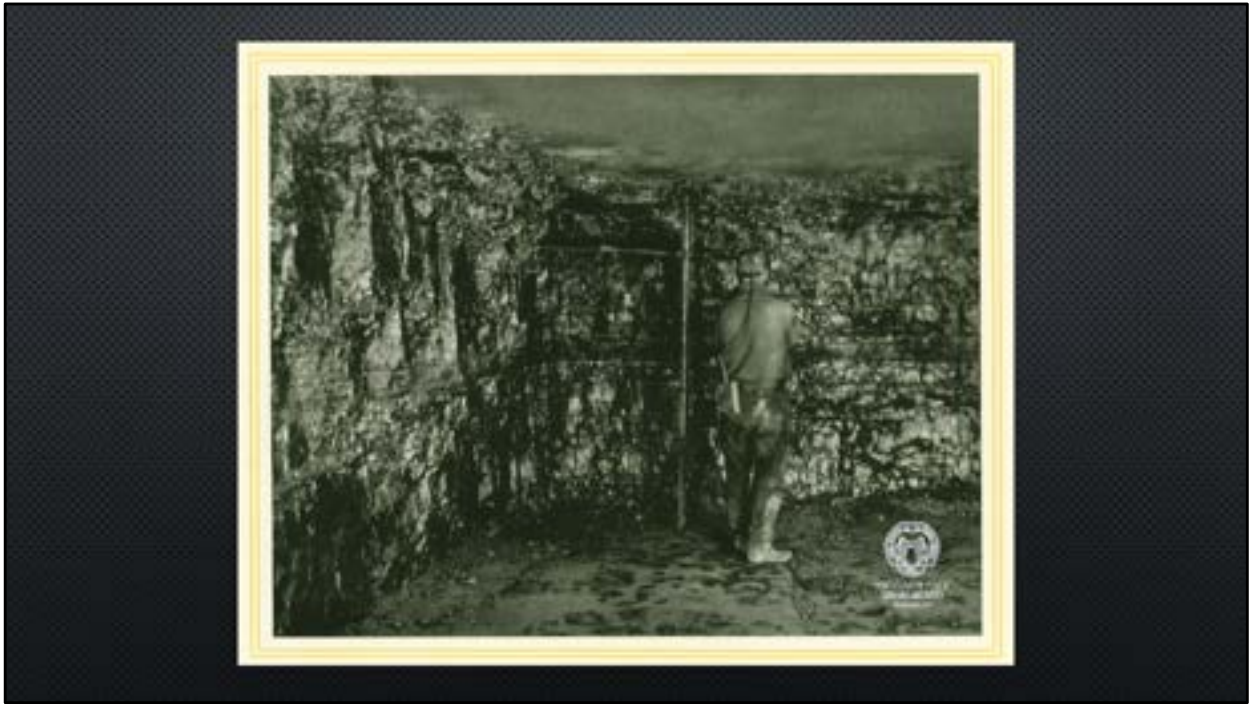
Here's a miner at work on a wall of coal. In Benwood this meant the Pittsburgh number 8 seam.
