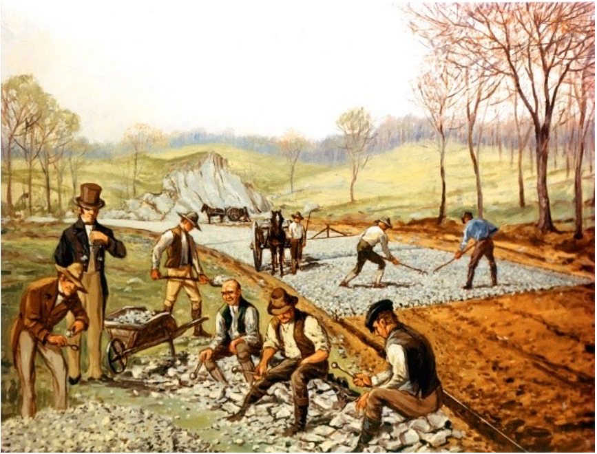
Workers building a section of macadam road on the Boonsboro Pike east of Cumberland, Maryland, ca. 1825 (courtesy Library of Congress).
