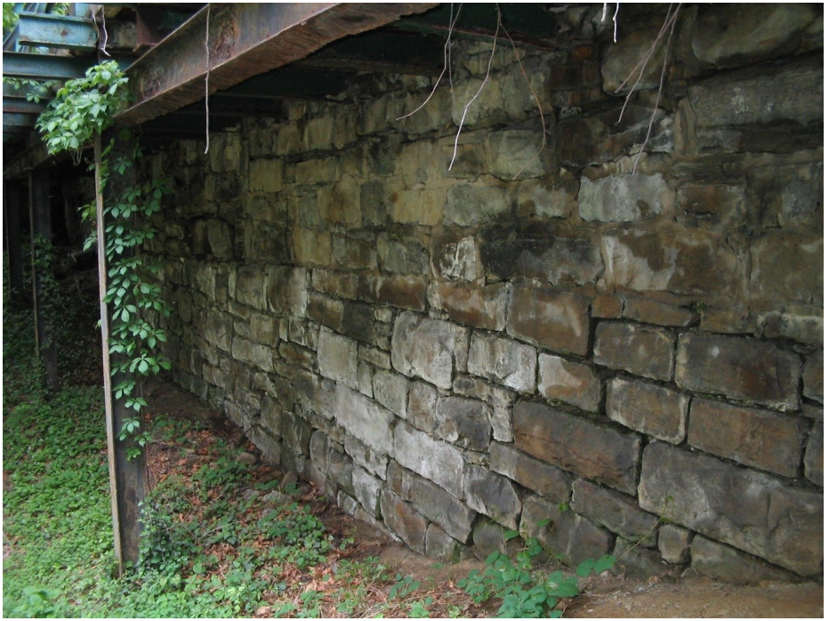
Figure 11. Stone sidewalls west of Elm Grove along the original alignment of the National Road.
